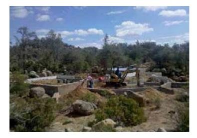
BEGIN FOUNDATION: AC Block (aerated auto-claved concrete) has been placed inside the foundation to insulate the home from the ground up creating an R-value of 10 for the underslab and a perimeter slab of R-15. The footings used high volume flyash concrete which reduced the use of Portland cement by 50% creating a more carbon neutral product. The insulation of the slab is critical to creating high energy efficiency but most builders, today, use minimal foundation insulation.
