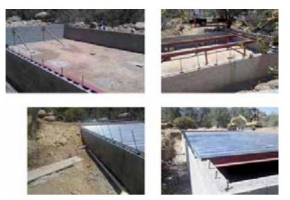
The upper left photo shows the excavation and foundation for the garage. The photo on the upper right shows the steel substructure required for the extra weight of parked cars. The bottom two photos show the steel deck covering the substructure. Concrete was then poured on top of the steel decking with access to the water storage area maintained.
