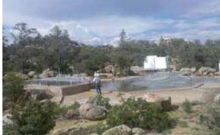
FOUNDATION POURED: The foundation is poured.... again using high volume flyash concrete that reduces the use of Portland cement by 50%. It will later be color etched. Along with the Poured Earth walls, these concrete floors add to the mass to store heat during the day in the winter and cool during the night in the summer.
