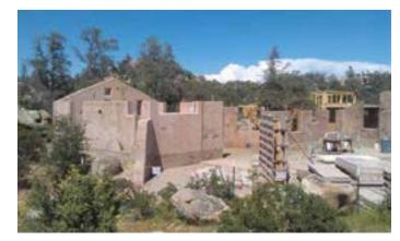
POURED EARTH WALLS: These beautifully colored Poured Earth walls are the first to make use of MgO (magnesium oxide) along with flyash to reduce the use of Portland cement by 50%. Because MgO sequesters more carbon than is used to make it, it moves Poured Earth technology one-step closer to becoming carbon neutral!
