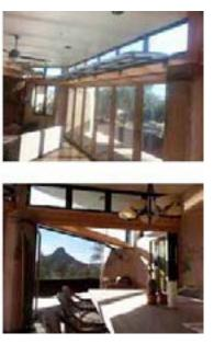
NANO-WALL EXTERIOR SLIDING DOORS: These bi-folding doors open the south wall dramatically to connect interior spaces to the natural landscape. They are certified to have very low air infiltration
