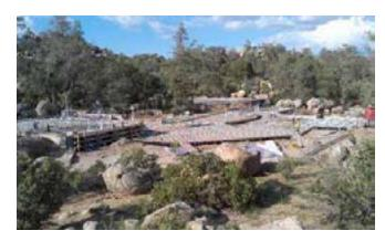
IN-FLOOR HEATING LAYOUT: Before the foundation is poured, the piping for the in-floor heat and cooling system is laid out. This system is the back up heat source for ultra cold, cloudy days and the means for delivering cooled water provided by night sky radiation during the summer -- an inexpensive means of "air conditioning." This system will be zoned throughout the house for full efficiency.
